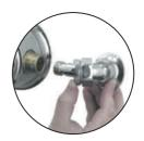
Carefully locate the elbows into the valve inlet connections and push fully home. Using the 2.5mm hexagonal key provided, tighten the locking screw enough to retain the elbows in the connections whilst still allowing ease of movement for final adjustment.
