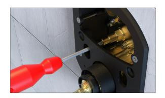
4. Open both built-in servicing valves (unwind – counter clock-wise).
