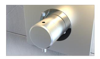
9. Insert the silicone cover cap, then open the water isolation valves and test.
