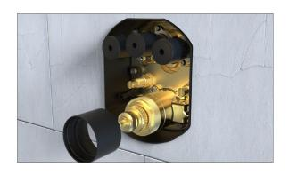
2. Install the dial shroud by rotating it onto the threaded headwork.
