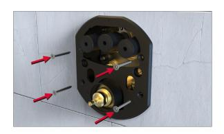
3. Install the compression plate using the screws provided.
