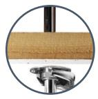
Cut off the excess pipe allowing for a suitable working length to allow for the required 22mm connection. If a push fit connector is to be used then the pipe must be abraded to remove all chrome plating.
