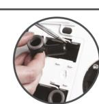
Screw in the two upper fixing screws leaving the heads projecting about 10mm from the wall surface. Feed the working end of the low voltage cable through the entry point in the back plate. Locate the back plate in position on the projecting screw heads. Ease the back plate downwards and engage the screws in the slots. Fix the lower fixing screw and tighten the upper fixing screws.
