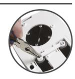
Lubricate the supply pipe ends using a silicone based lubricant and carefully slide the Aquastream  $^{\text{™}}$  Thermo unit onto the pipes whilst feeding the low voltage cable through the cable entry point. Secure the unit to the wall using the screws provided (if suitable). Proceed to step 17.
